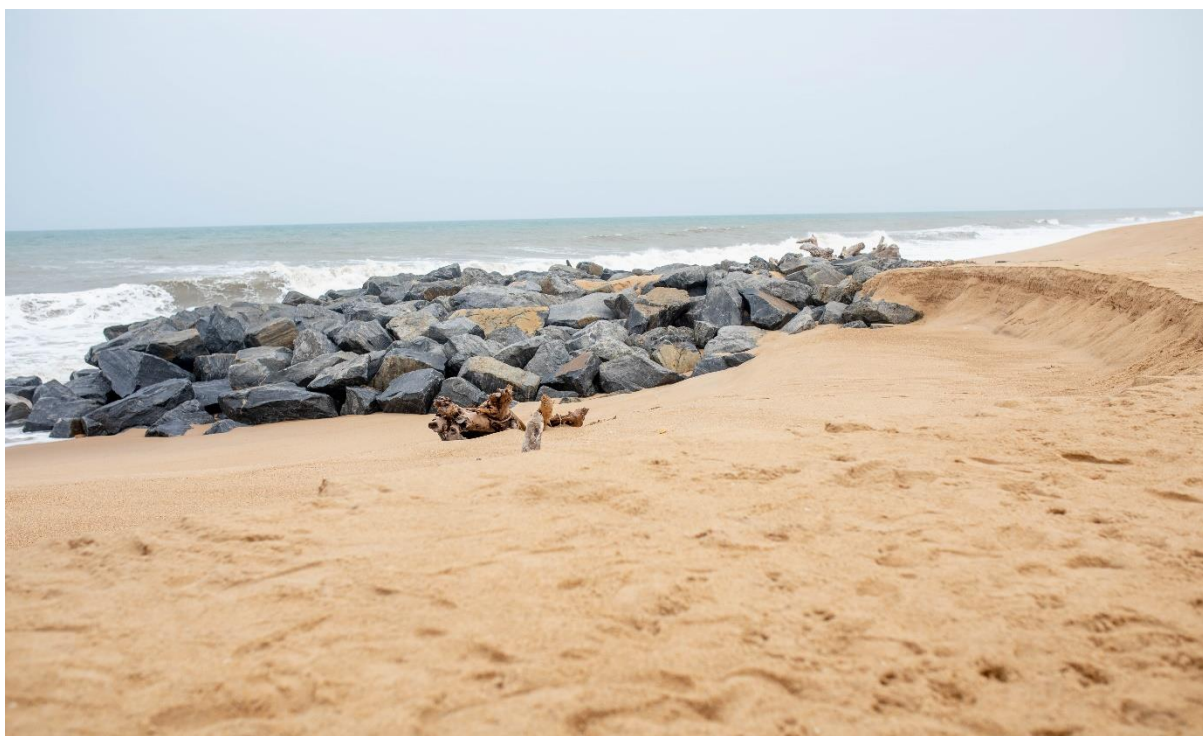
A coastal protection structure observed during the field visit
