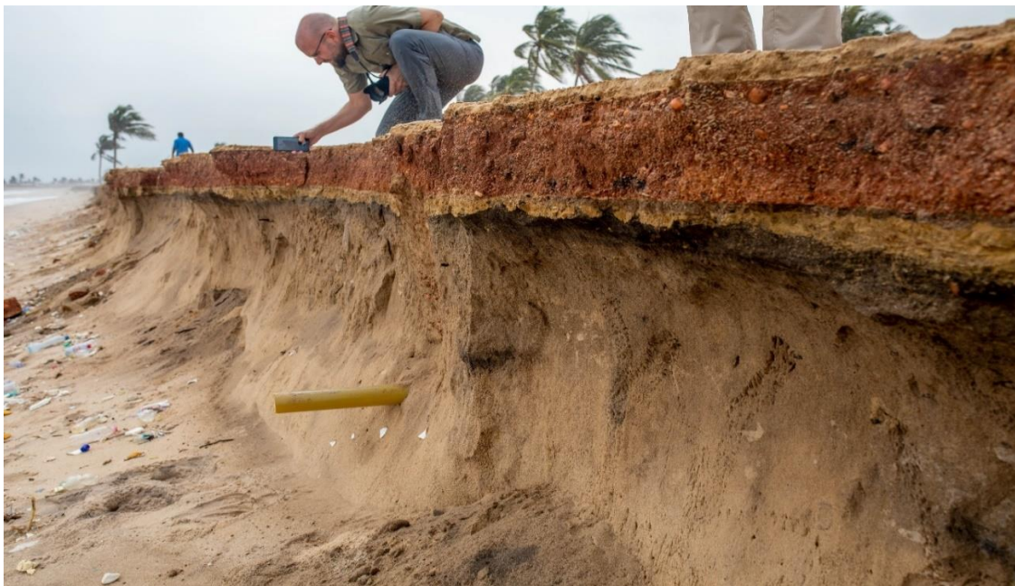
A picture showing erosion along the coastline
