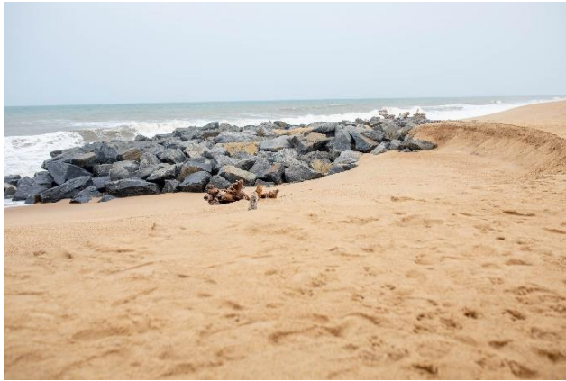
Fig. 14 Sea defense structure at Akplorwotorkor in the Anloga District of Ghana
